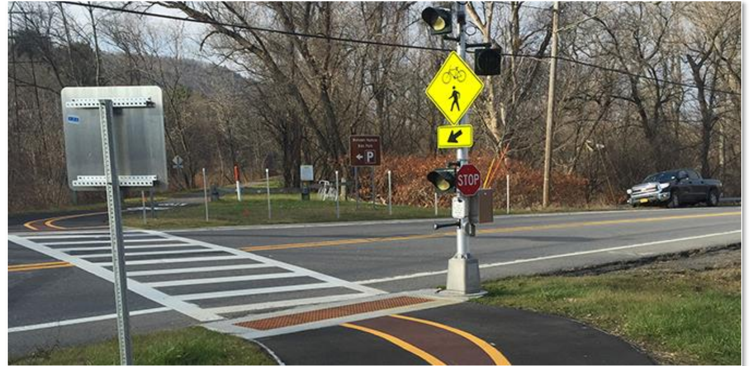
Wide, Painted Trail Crosswalk
