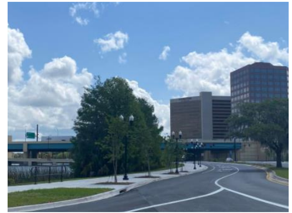
Countermeasure #18 (South): To the south of Poinsettia Avenue, the trail runs along Ivanhoe Boulevard. This image shows the wide sidewalk that the City of Orlando built along this section of trail in 2022 during the late development stages of this report. This was previously a countermeasure area.
