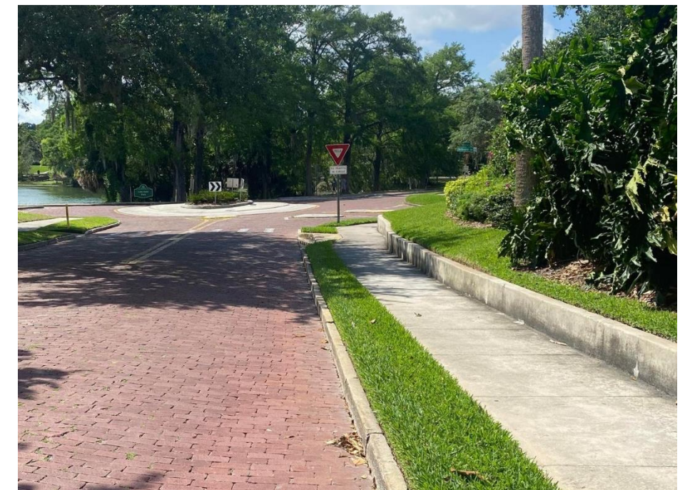
Countermeasure #17A: This trail segment would be adjacent to the roadway at the Lake Adair Boulevard intersection. If warranted, the curb could be extended inward toward the road in order to provide 10-feet of space for the trail. Thinning the trail to 8-to-9-feet in this location is also an alternative.
