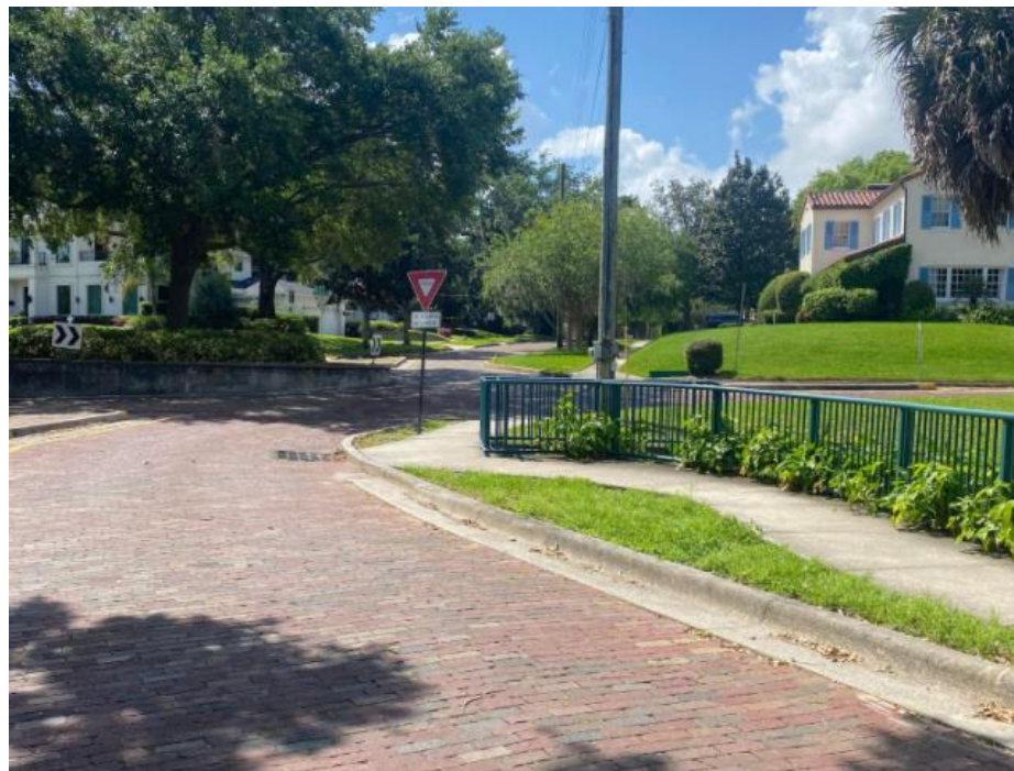
Countermeasure #17B: Located at Edgewater Court and Westmoreland Boulevard, this project would reduce the width of the right turn lane in order to add more width to the trail. Alternatively, the trail could be reduced in size to 7-to-9-feet in this location.
